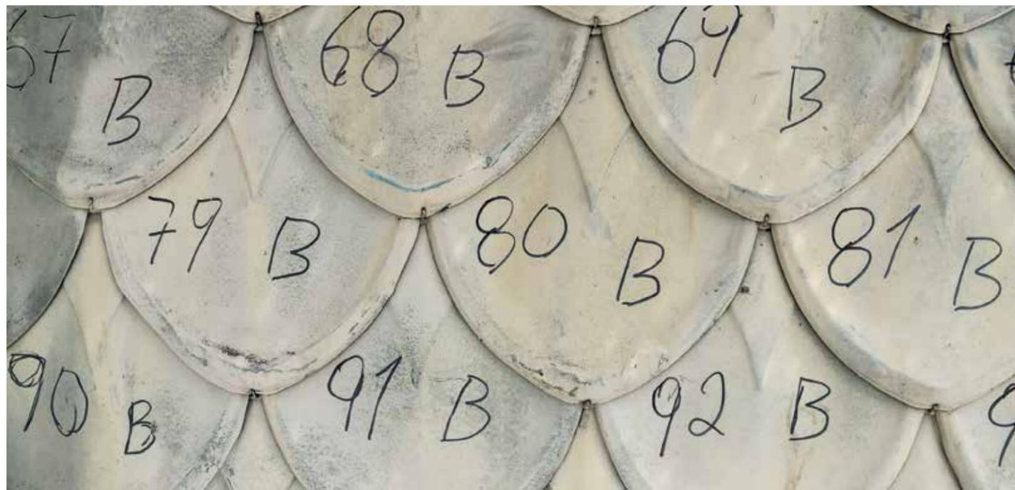
Once the scaffolds were in place, the petals, ornaments and other copper pieces were painstakingly mapped out. They were then removed, labelled and numbered.
